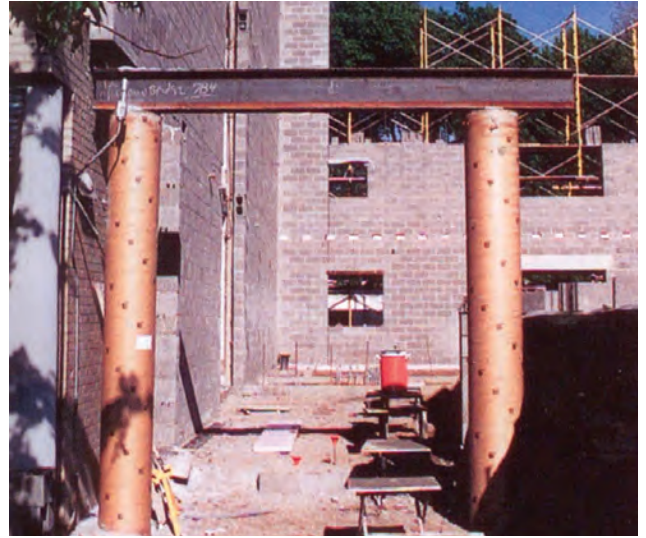
Walls of the new south wing construction going up.
